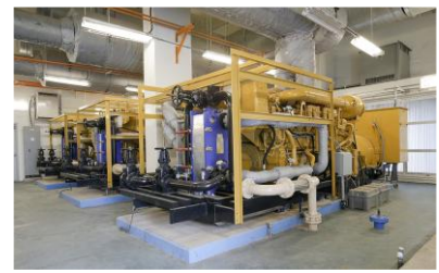
(c)大型应急发电机组
